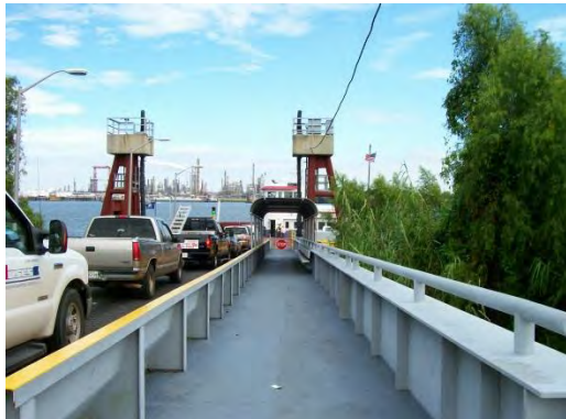
Lower-Algiers Landing, Vehicle and Pedestrian Approach, 2008
