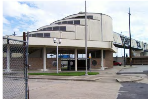
Jackson Street Ferry Terminal, Pedestrian Bridge, 2008
